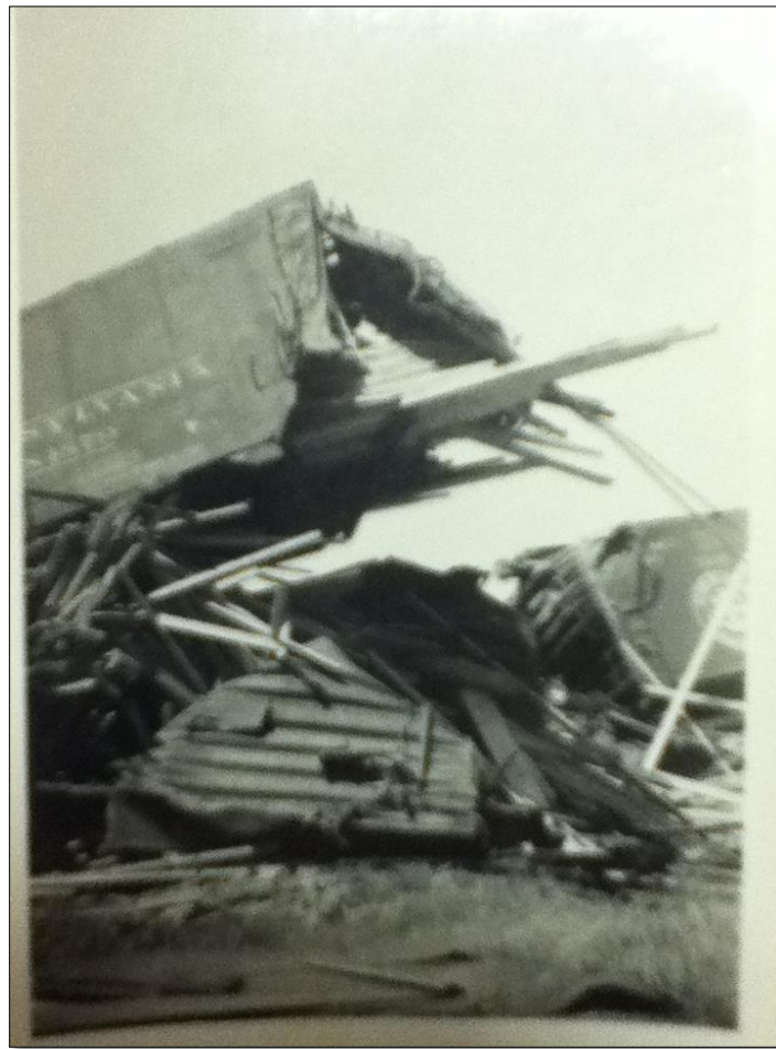
Figure 10. A photograph of the train wreck in Langley, 1952, clearly shows that the cars were transporting lumber. Photograph provided by Charlotte Koehn.
