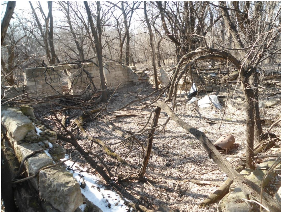
Figure 2. Mill site foundation at Alta Mills. April, 2013. Photograph by Grant Peters.
