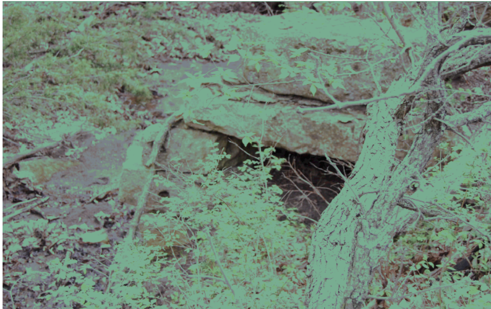
Figure 1: Photograph of the remnants of the stone bridge. SOURCE: Photograph courtesy of Jim and Marian Bradley.
