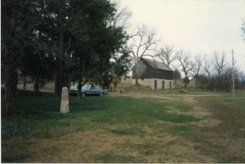
Side view of the barn on Middle Creek farm, Marion County, October, 1985. Notice how the barn is made up of two different materials: wood and limestone. According to the present owner, the stone foundations are still visible today on several out buildings. Also, notice the stone post resting in front of the trees. It is believed that this is an old hitching post. Photograph courtesy of Barbara Booth.
