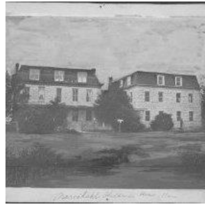
Figure 4: Mariadahl Children's Home after renovations; undated
