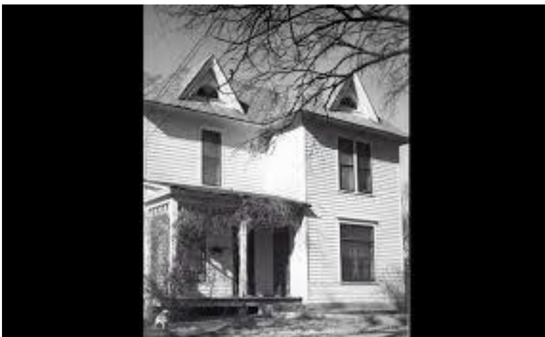
Figure 1. Photograph of the Porter Morgan Hospital, the first hospital in Clay County, Kansas. Photo courtesy of Clay County Medical Center: http://www.ccmcks.org/ourhistory1920.php
