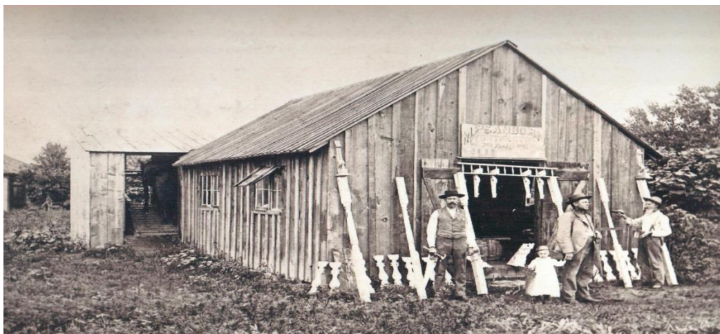
Figure 1: First Carpenter and Contracting shop (opened in 1892) built and owned by Malte Persson Sanborn. SOURCE: Malte P. Sanborn Family of Chapman, Kansas .
