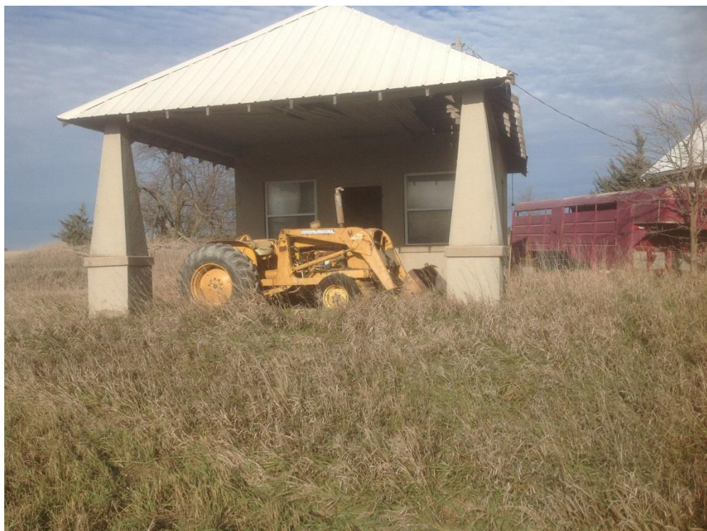
Figure 4: Parallel Filling Station
