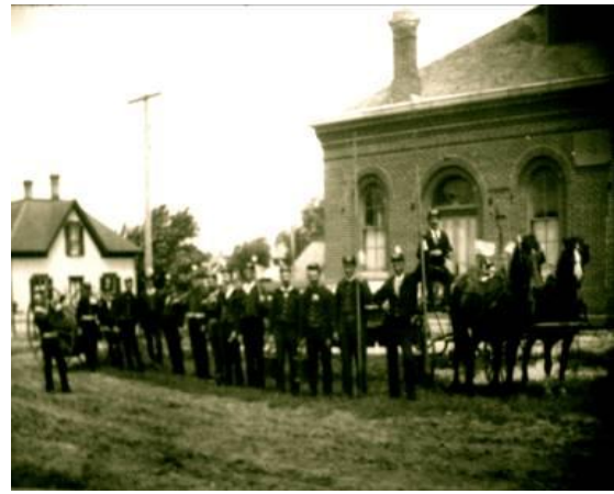
Figure 20 Fire Company 1886- Turner Hall in Background (W.C.M.)
