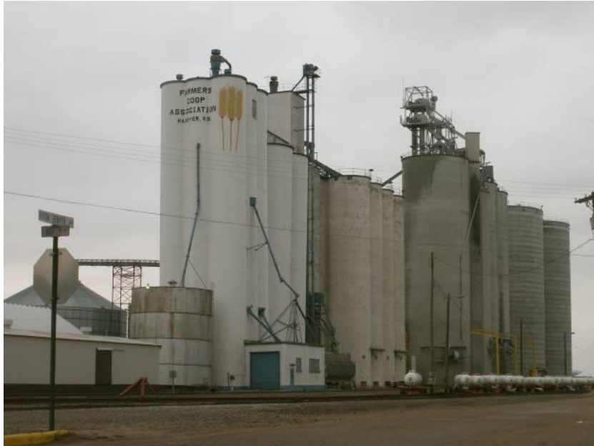
Figure 6 Hanover Elevator 2/28/2012, Hanover KS
