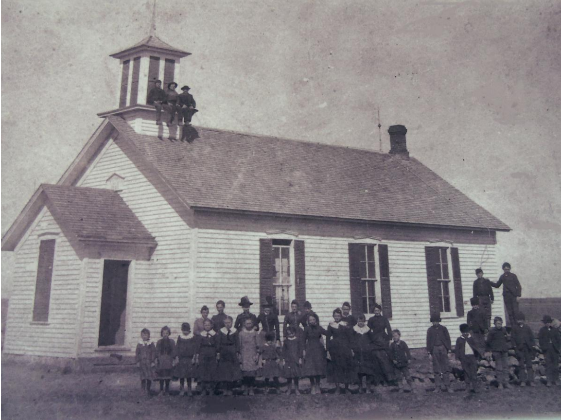
Figure 4. This is a picture of the Emmons schoolhouse, circa 1890s, after the community added a steeple and an entrance.
