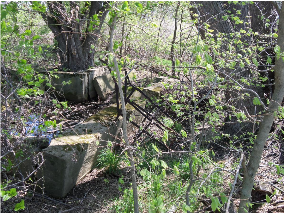
Figure 5. This is a photograph of the foundation of the General Store in Emmons. Source: photo taken by the author.
