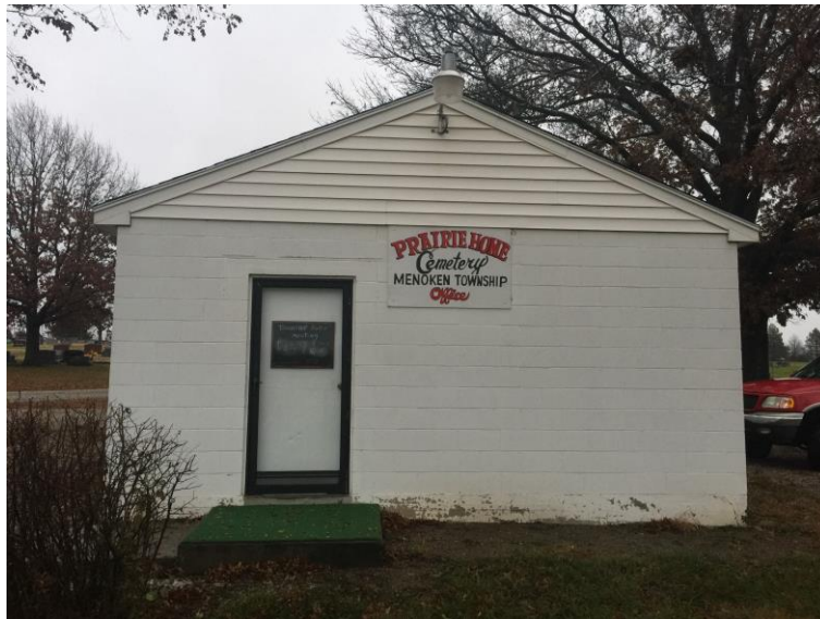
Figure 2. This photograph shows the office building of the cemetery that currently resides in Menoken Township on Menoken Rd. SOURCE: Photo taken by Nicholas Gonzalez 2015
