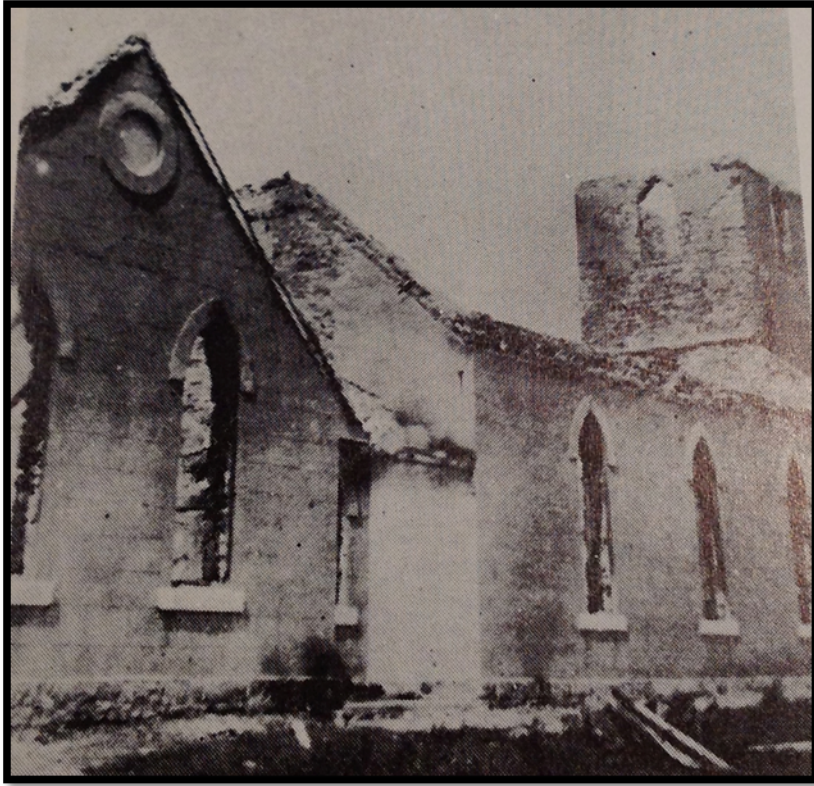
Figure 10. Photograph of the church after the lightning strike ca. 1918. The stone walls were all that were left after the fire. Photo from Walsburg Lutheran Church, Leonardville, Kansas, 1873-1973 .
