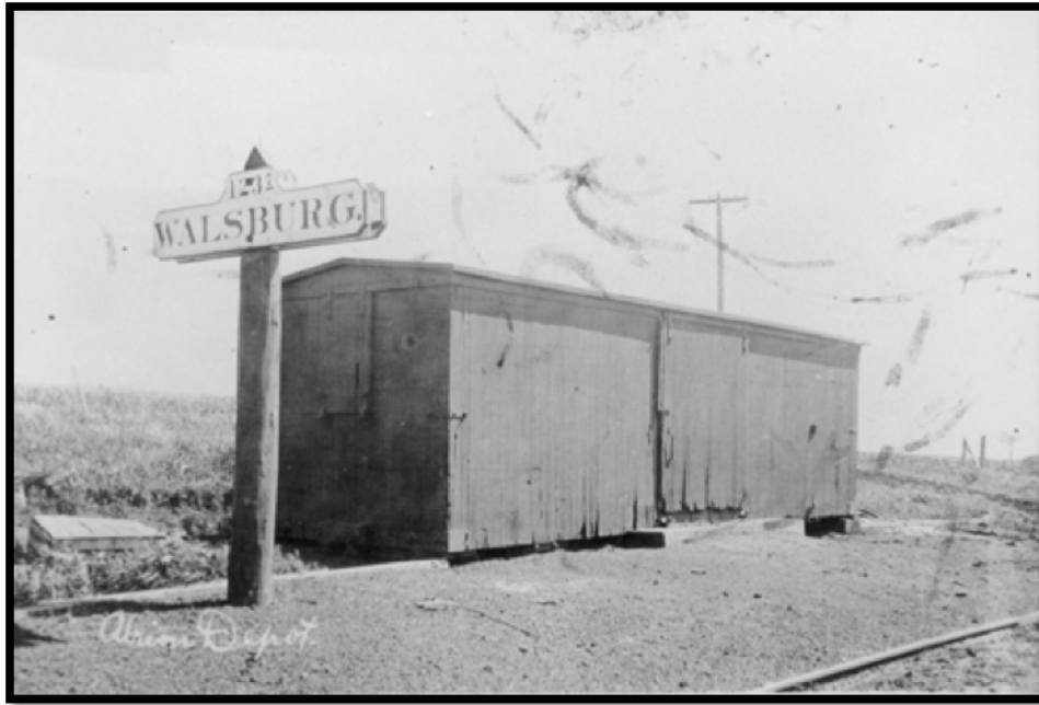
Figure 4. Photograph of Walsburg Railroad Depot ca. 1930. The depot in Walsburg was housed in an old boxcar; notice how temporary the depot appears. Photo courtesy of Riley County Historical Society.
