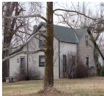
Figure 2 John Locke house, Riley, KS. Dec. 2, 2010. The limestone portion of this home was built by Mr. Locke and his sons. Which they removed from Wildcat Creek that is located near the property. They used stone since it was readily available and lumber was not. This was also one of the earliest permanent dwellings built at Riley. SOURCE: Photograph taken by author
