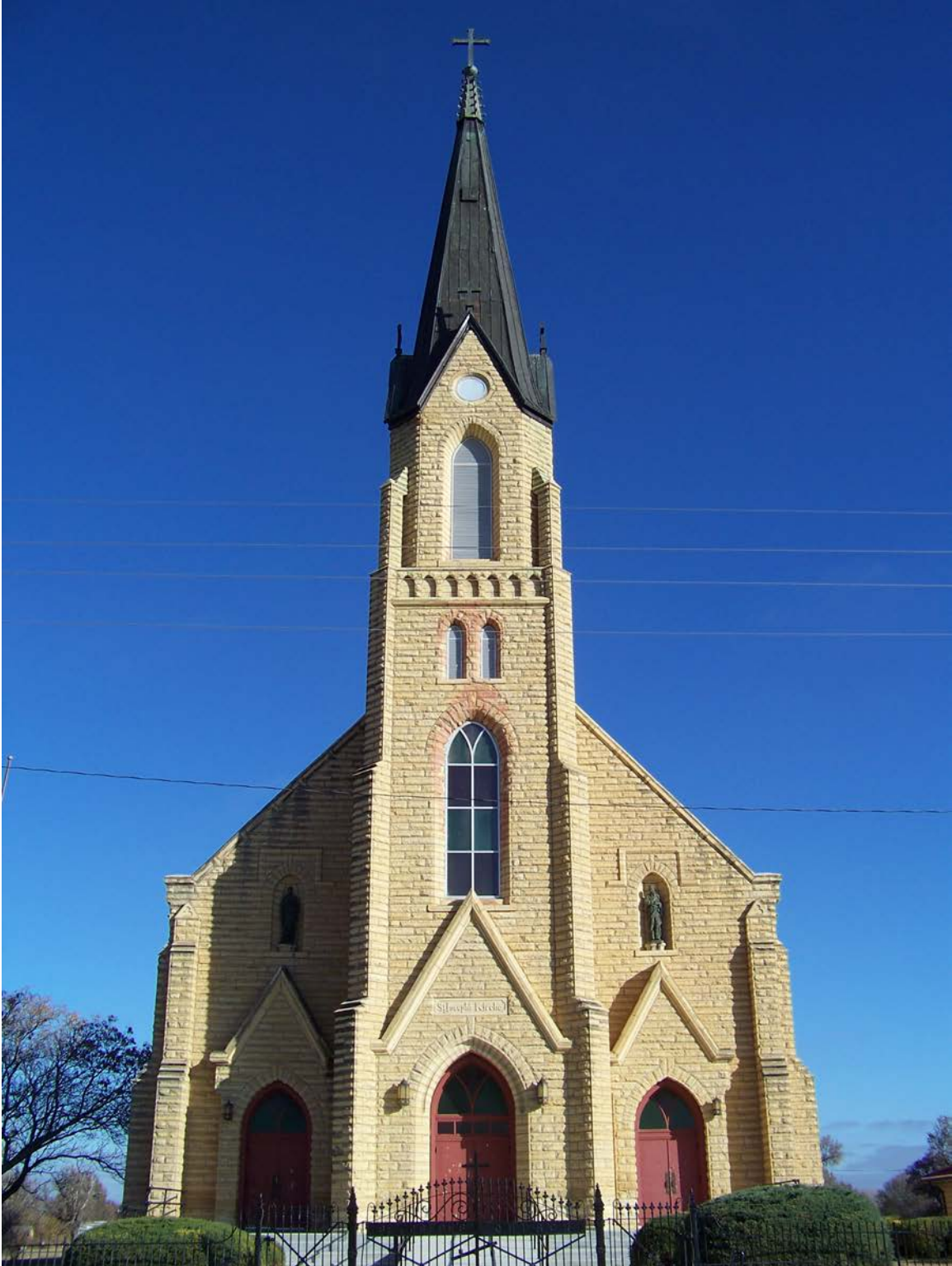
Figure 12: This photograph shows the beautiful limestone church, St. Joseph's Kirche. This church has miraculously survived 2 fires since its completion in 1905.
