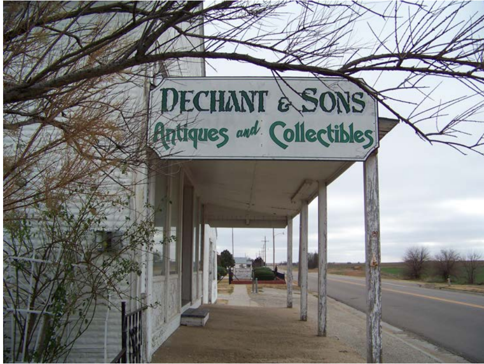
Figure 11: This photograph shows the Dechant and Sons Antiques and Collectibles. This building was formerly Dechant Grocery, and Herrman's General Merchandise Store. This building was saved in the fire of 1917.
