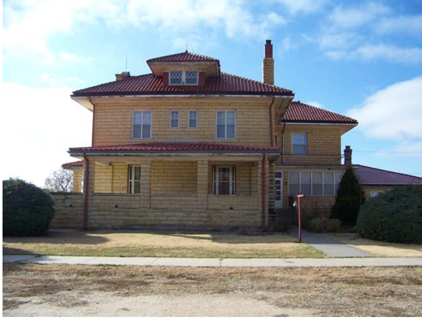
Figure 17: This photograph shows the exterior of the church rectory's east facing entrance.
