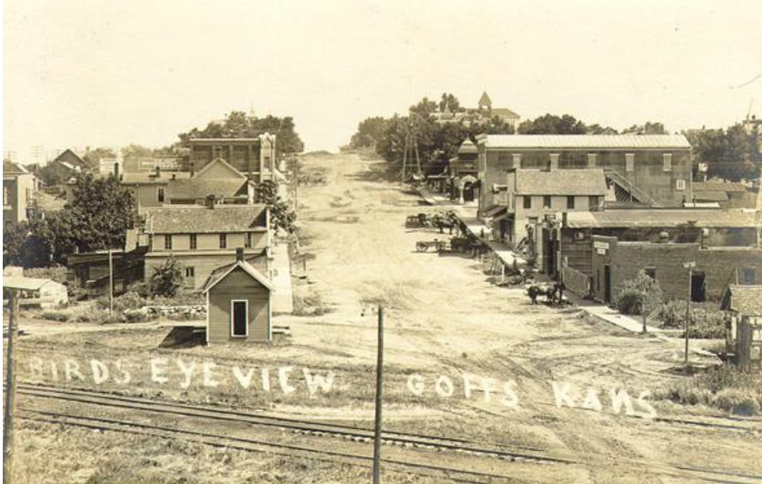
Figure 1. Photograph of a bird's eye view of Goffs (sic), Kansas, looking north on Stahl Street, c. 1905. Today, the bank on the corner of Stahl Street and Second Street (now Highway 9) is the only remaining original structure, including the railroad tracks, seen in the photograph. SOURCE: Special Collections and University Archives-Wichita State University Libraries
