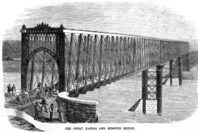
Figure 2: The Great Kansas and Missouri Bridge from the March 1873 issue of Scientific American . The stone abutments in the water were built from Bigelow area limestone. Source: http://bridgehunter.com/ks/leavenworth/fort-leavenworth/
