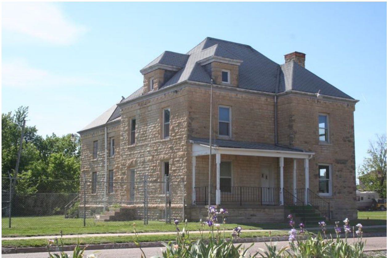
Figure 4: Photograph of the former Washington County Jail in Washington, Kansas Circa 2011 This Jail was made from Bigelow Limestone built in 1899. It is listed on the National Historic Register. Source: http://www.kshs.org/kansapedia/james-c-holland/16802
