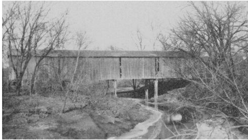
Figure 2. A black and white photograph of the Jarbalo Bridge, crossing over Stranger Creek. Its modern equivalent can be found one-mile north and one mile east of Jarbalo. This photograph was taken sometime during the 1930s. SOURCE: kansasmemory.org.
