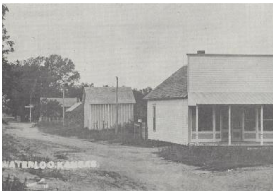
Figure 1. A photograph of Waterloo stores and post office c. 1910. This photograph was taken looking south on Main St., now known as NE Waterloo Ave. None of these buildings stand today. SOURCE: Waterloo - Galesburg Township Kingman County, Kansas by Irene Bergkamp
