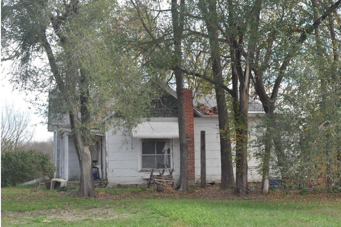
Facing east, an abandoned home on Central Street.
