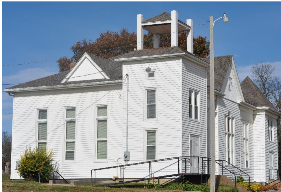
Figure 15. A photograph, 2016. Denison Reformed Presbyterian Church has met in the same building since its construction in 1884. Its large steeple has been replaced with a lower, sturdier structure. Photograph by author, 2016.
