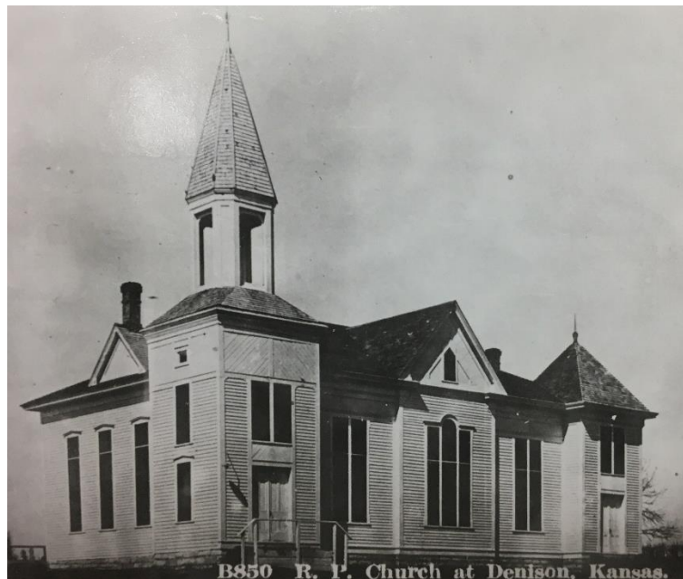
Figure 9. A historic photograph, c. 1885. This structure was built for the Reformed Presbyterians in 1884, after a vicious windstorm blew down another conception of this building in 1883. Almost $2,500 was raised for its construction. SOURCE:
