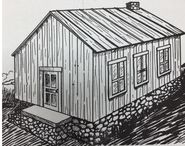
Figure 8. A historical sketch, c. 1871. This was the “Tabernacle” built by the Reformed Presbyterians, or Covenanters, in 1870. It was built of native lumber and had a dirt floor covered in hay; all in all, the building cost was $185.95 and measured 45x63 feet.
