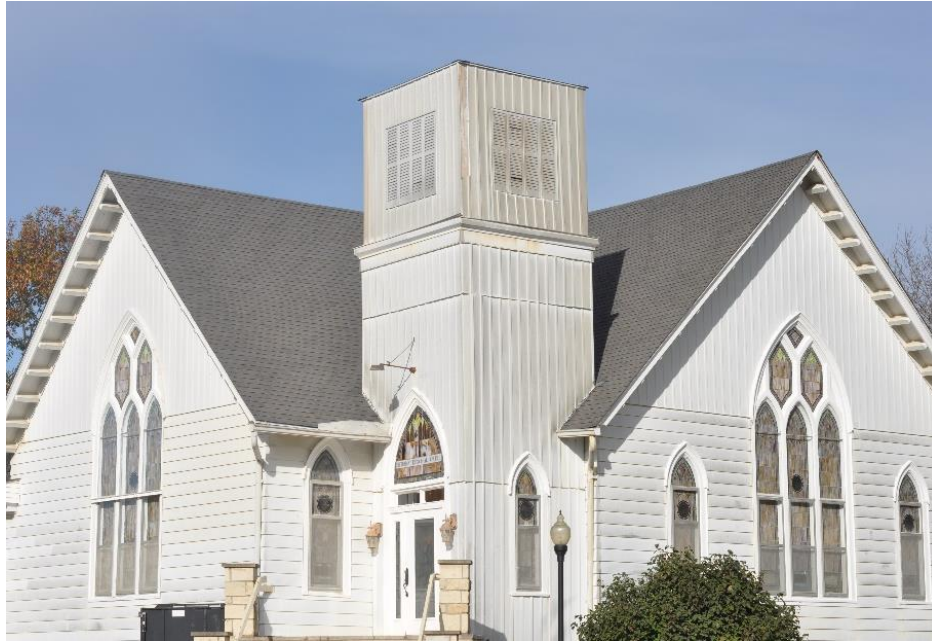
Figure 14. A photograph, 2016. The Denison Bible Church still occupies the Methodist Church building, having added on to the west (left) side of the structure with more classroom space. While the bell tower doesn't look as ornate, it does still sit in the belfry, ready to be rung. Photograph by author, 2016.
