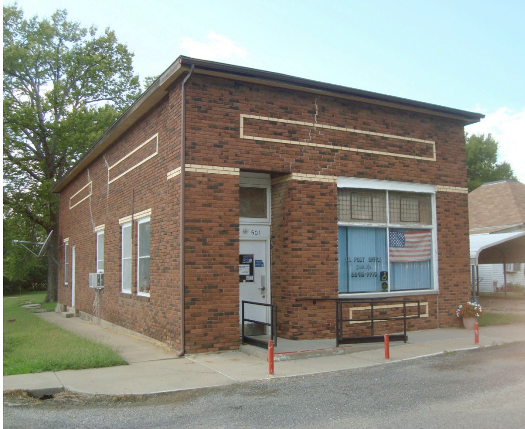
Figure 1: Former Delia State Bank, current Delia Post Office
