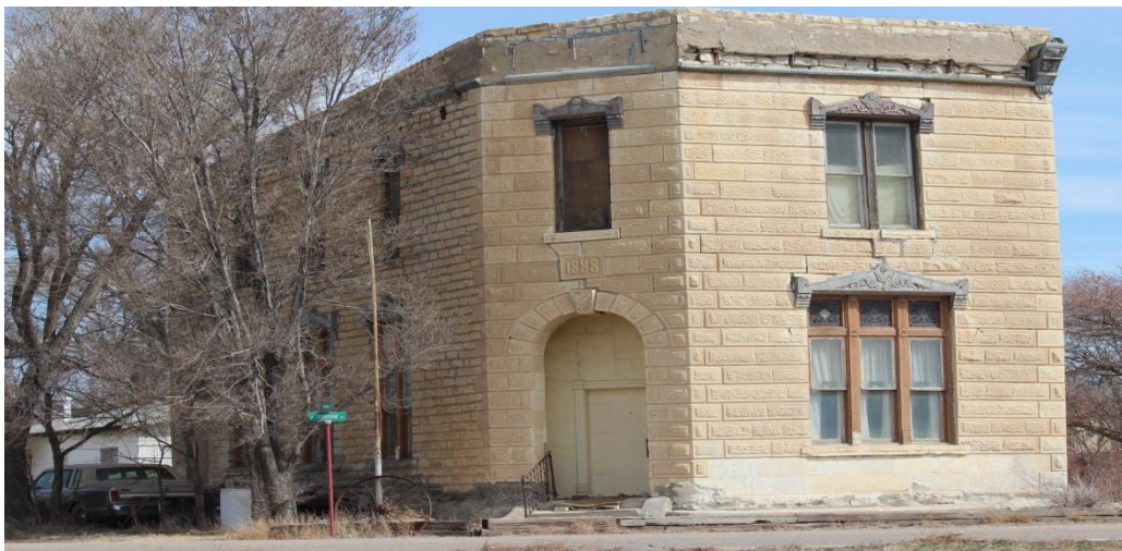
Figure 3. 8 This building was constructed in 1888 along what is now Highway 50 and was the home to the Coolidge State Bank, which moved here in that year. The stone architecture of this bank is very similar to what you see in many small town banks all over western Kansas, with a corner front entrance for protection. Photograph by author, March 16, 2013.
