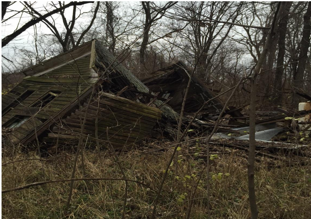
Figure 2. A photograph of Mary Ann Roundy’s house. A fire destroyed it in 1884 and then it was rebuilt to what it now looks like. Located to the north side of Geary City. Source: Photo taken by the author, Dec. 15, 2015.
