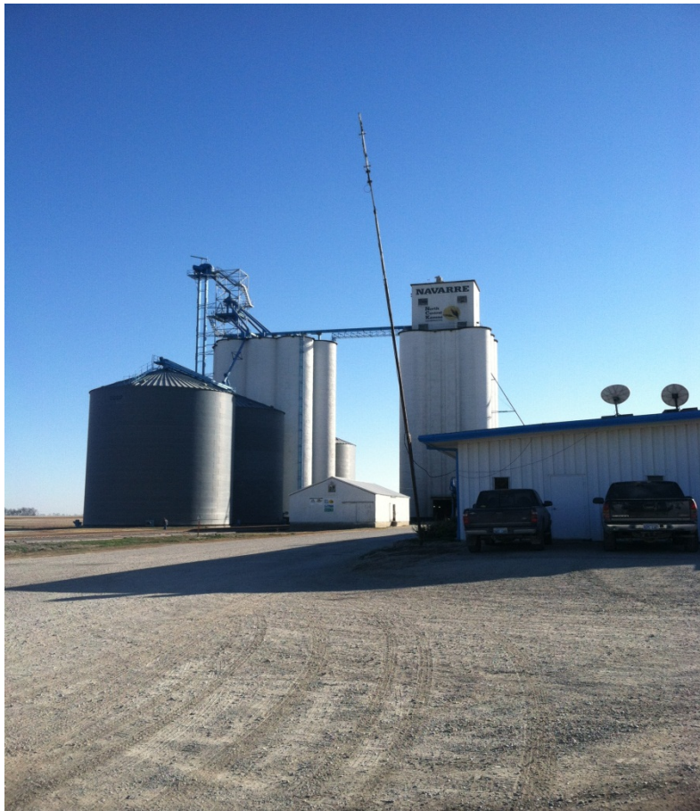
Figure 8. NCKC elevator on the south side of Main Street. Photograph taken by Adam Coup, December 8, 2012.
