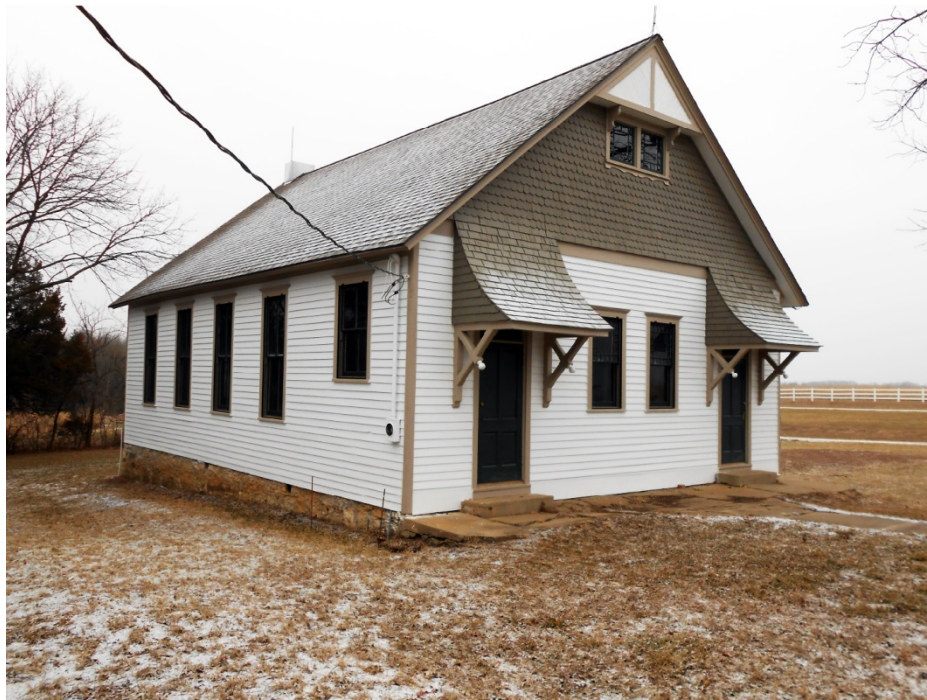
Figure 6: The Clearfield School which is currently under renovations. ca. 2013 SOURCE: Author
