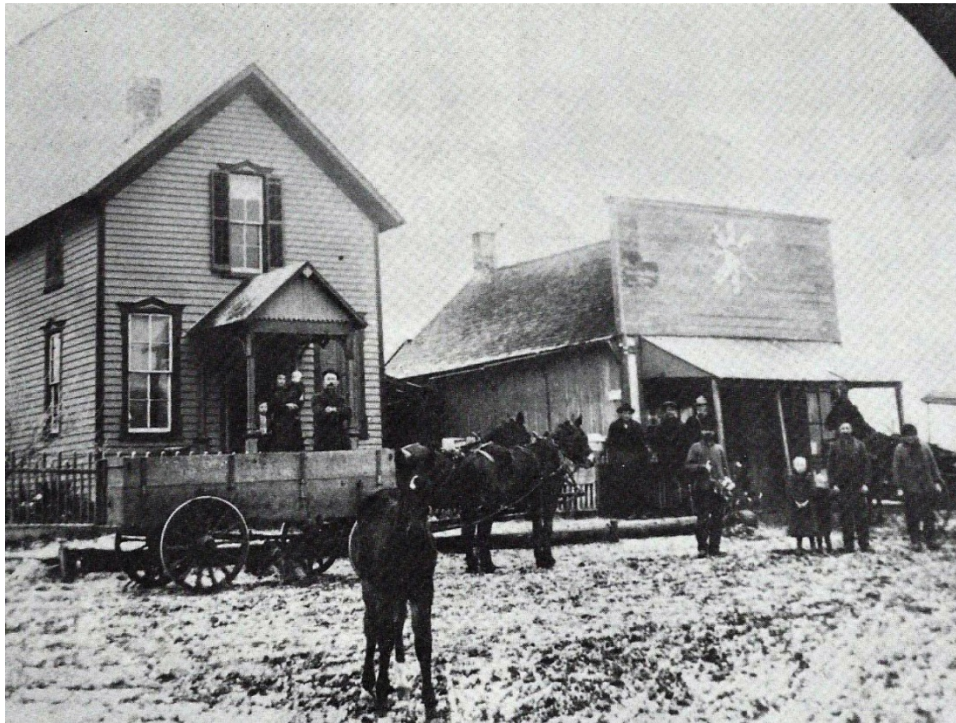
Figure 8: Scanned photograph of the Clearfield general store and post office. ca. 1900 SOURCE: Clearfield History 1858-1976 , 13.
