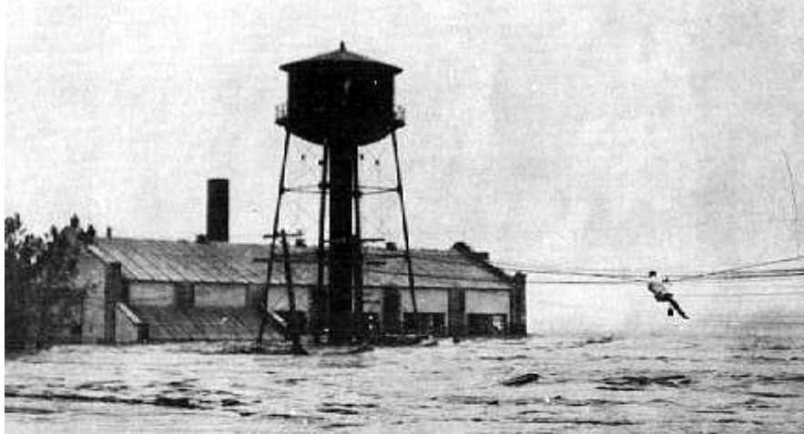
Figure 2: Photos demonstrating damage from the repeatedly flooding Republican River which caused the eventual undoing of Sherman. It was not economically feasible to keep rebuilding every time the river folded. Circa 1930s.
