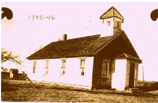
Figure 4 Gatesville school 1945-46. This building was built in 1884, and was an unusual school building for the area as it was made of stone. This demonstrates the importance of the school to the community. SOURCE: Clay County Historical Museum.
