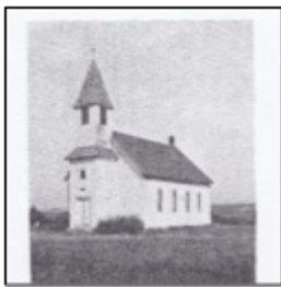
Figure 2: The original church built in 1905. Bethany Church, Clay County, Kansas
